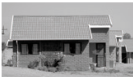
40m 2 unit with concrete tiles, ceilings, guttering and fascia boards
