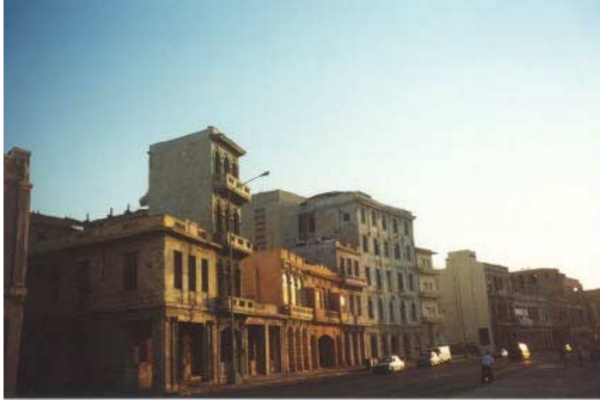
Housing located along the Malecon in Havana. This waterfront property, while poorly maintained, is a prime target for private sector development.
