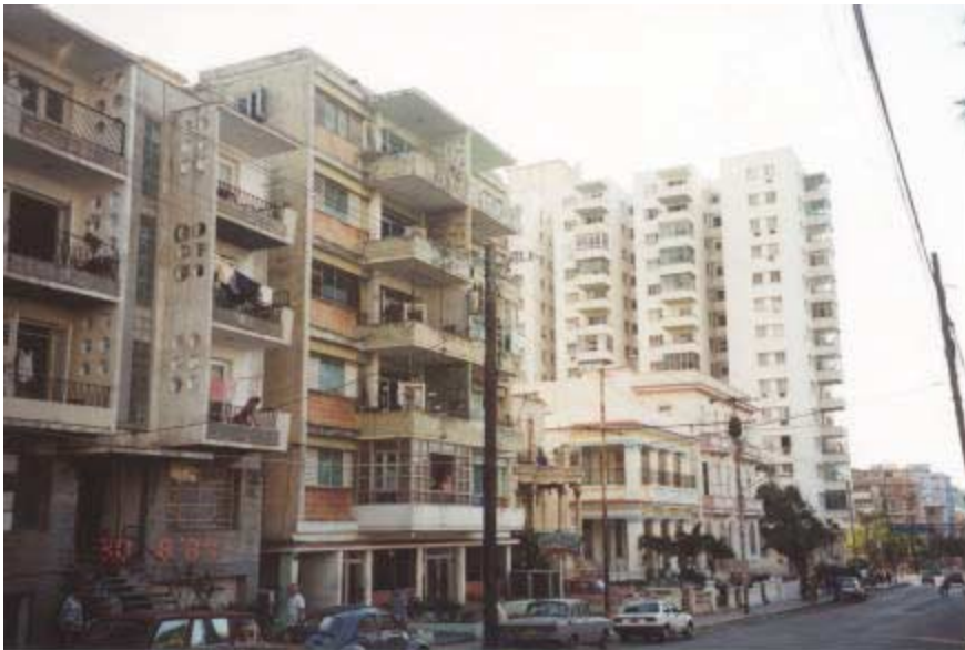
A mid-size apartment building in Havana. Signs of deterioration can be seen.
