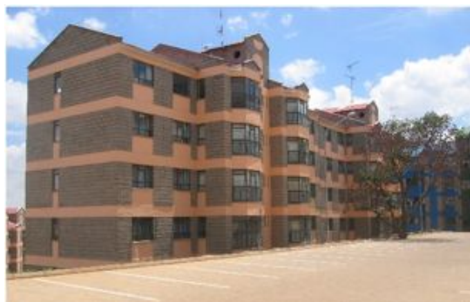
NHC high-rise flats in Langata
